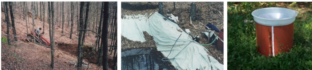
Fig. 3. Construction of the ditches, the pumping of surface runoff from the collectors and a collector of through fall (c, left) [8]
